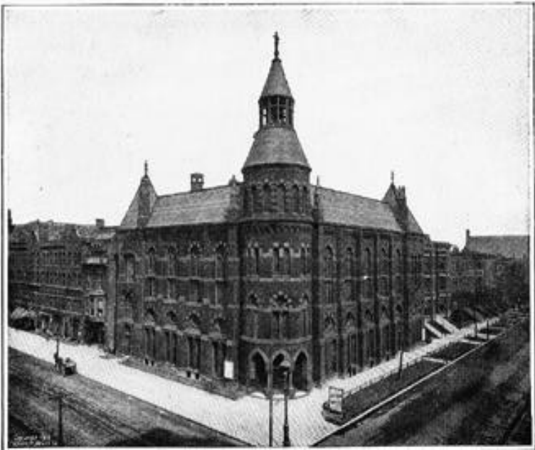
CHICAGO AVENUE CHURCH, CHICAGO. Buildings of Ladies' Department, Bible Institute, Adjoining at the right
